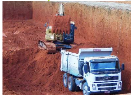
Paragominas bauxite mine Taking over 60%, increasing to 100% by 2015
