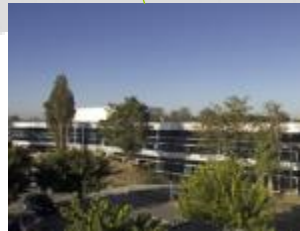
Technal Brand Development Centre, Toulouse in France
