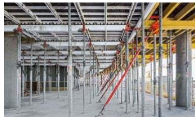
Aluminium formwork for B&C
