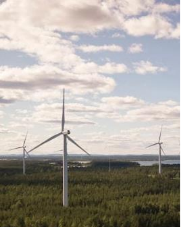
Renewable power in new areas: 60-70%
